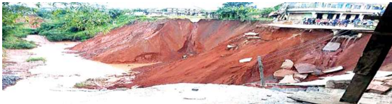
Figure I: A typical gully site in Southeastern Nigeria
